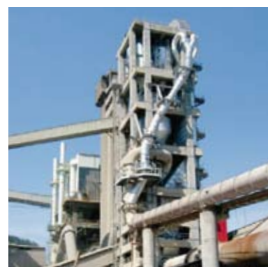
CEMENT WORKS, Spain PREHEATER KILN
