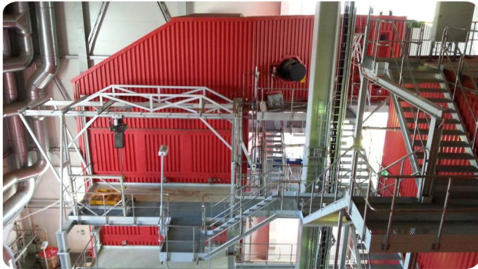
Woodchip stove, Sweden DeNOx
