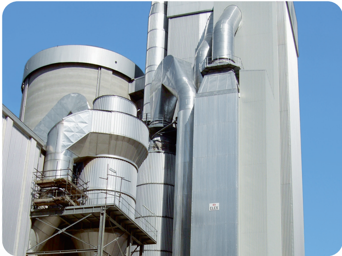
Cement works, Italy
