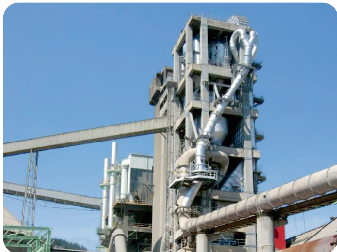
Cement works, Spain Preheater kiln
